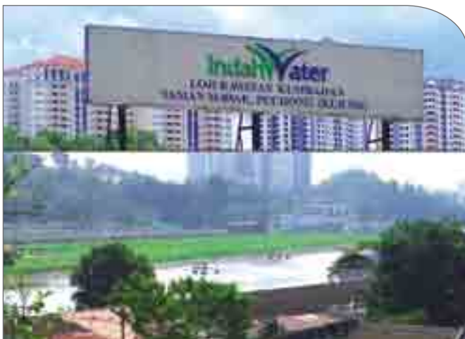
National Sewage Treatment Plant
