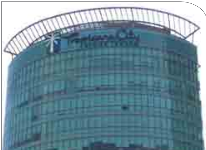
Tropicana Office Tower
